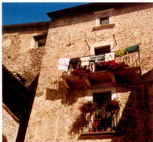
A ground-floor room. Above: a resident's laundry
